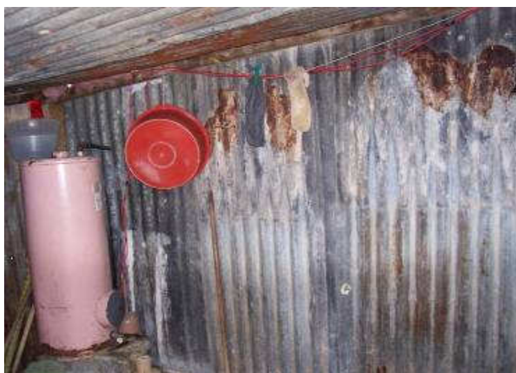
All-zinc shelter providing insufficient protection against the weather
