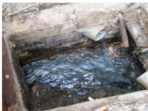
Underdimensionned manhole
