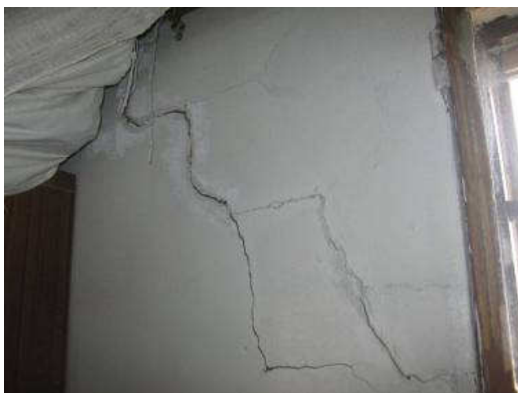
Diagonal crack in masonry (symptomatic of major structural problem)
