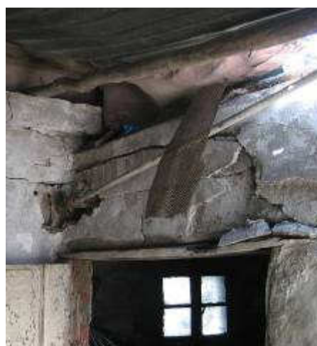
Cracked concrete lintel
