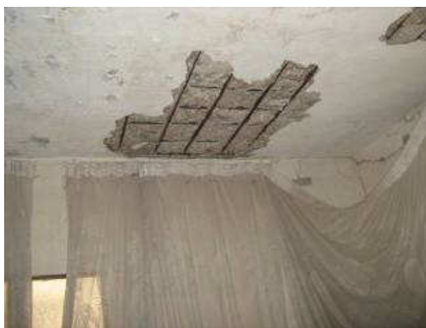
Damaged concrete roof, rusting reinforcements
