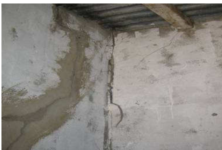
Crack in masonry
