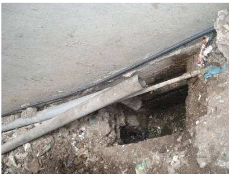
Uncovered inspection chamber, crossed by with water supply pipes
