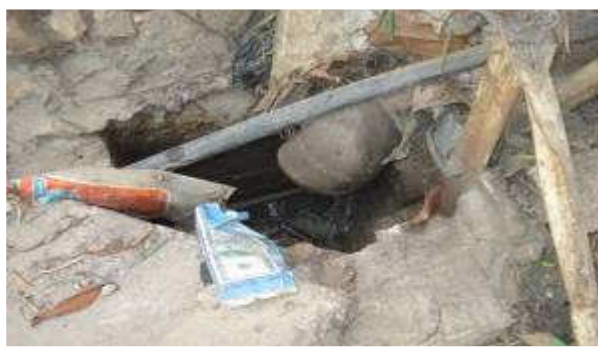
Damaged manhole crossed by water supply pipe
